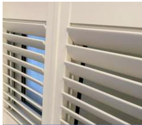
Concealed rod design - slats must close upwards.
