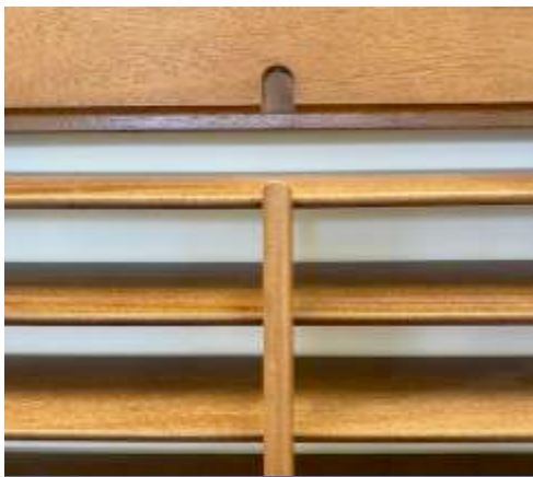
The hole for the Push rod is at the top of the panel.
