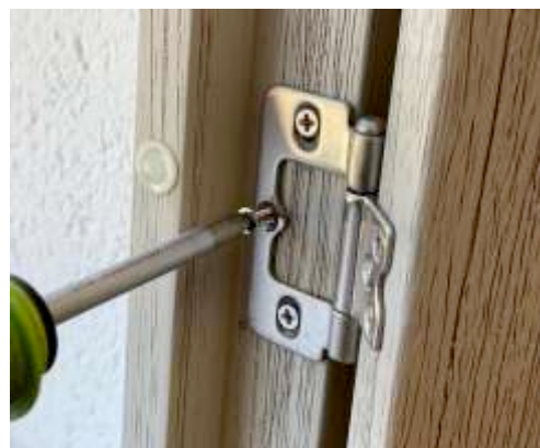
Final fix of screw in shutter hinge
